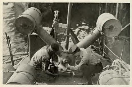
Depth bombs and Y gun on stern of a submarine chaser. The bombs, loaded with 300 pounds of T. N. T., are projected from the Y guns and the charge is fired by a hydrostatic device which can be set for any depth of water.
