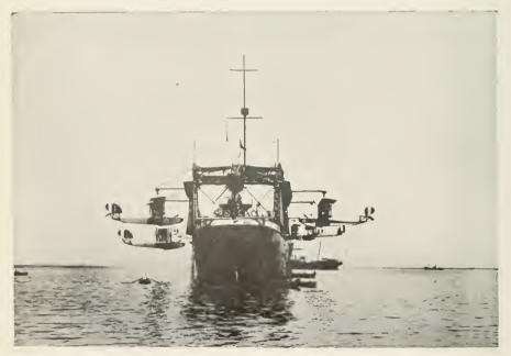
Italian scaplane mother ship. The seaplanes when at rest are carried on the ship and when a flight is to be made are lowered to the water.
