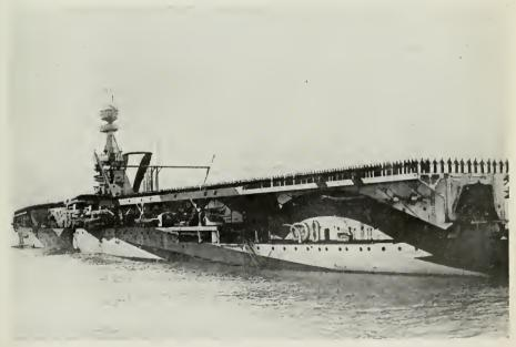
The British ship Furious, a "hush" cruiser, "dazzle" painted, used as a floating aerodrome. The ship is covered with a long, broad platform upon which the aeroplanes start and alight.
